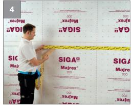
• Seal overlap with Sicrall avoiding tension and wrinkles
