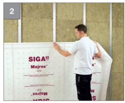
• Apply vapour control layer with the writing facing you **press firmly onto Twinet 20**
