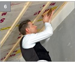
Paste over injection hole using Signal 170
