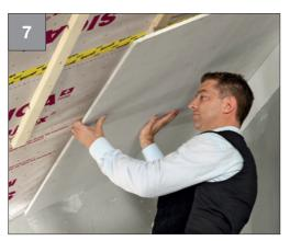
Finally install interior cladding (protects against mechanical influences and UV radiation)
