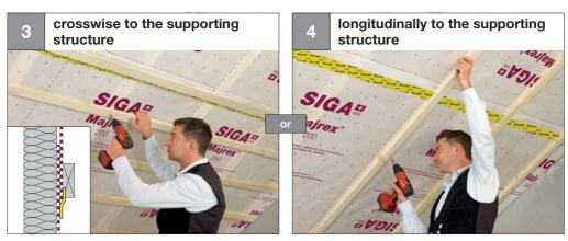
Before injecting the insulation material:
