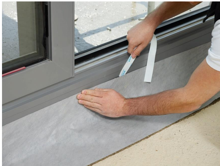
Figure 4 Removal of release film
