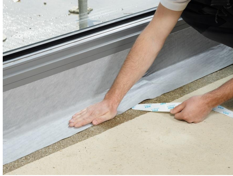
Figure 5 Removal of remaining release films, applied tension free
