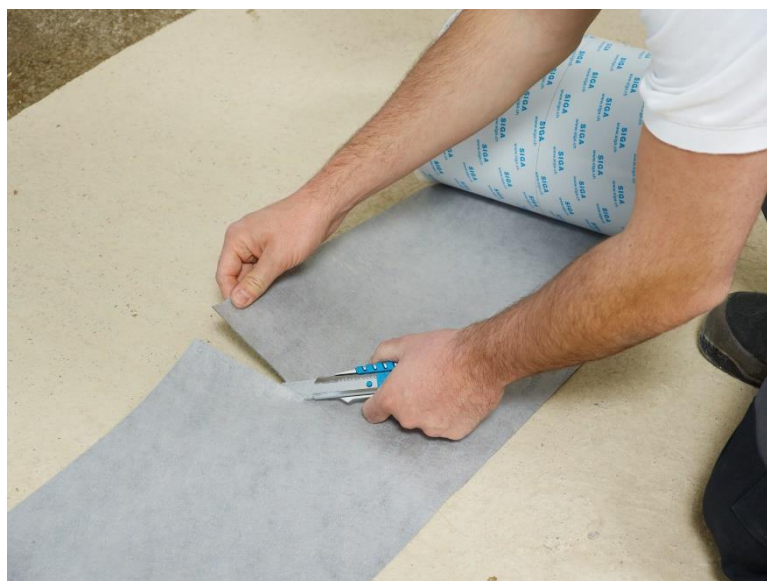
Figure 2 Cutting membrane to length
