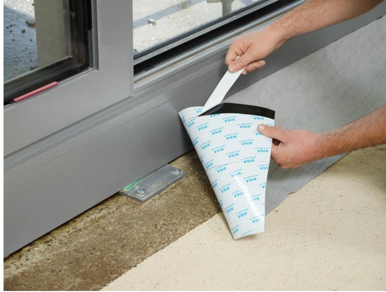
Figure 3 Starting removal of release film
