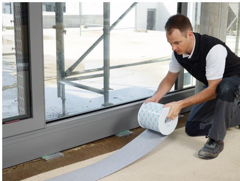
Figure 1 Laying out membrane
